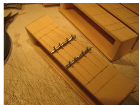
Fig. 19. Truss rods and queen posts in final position.
