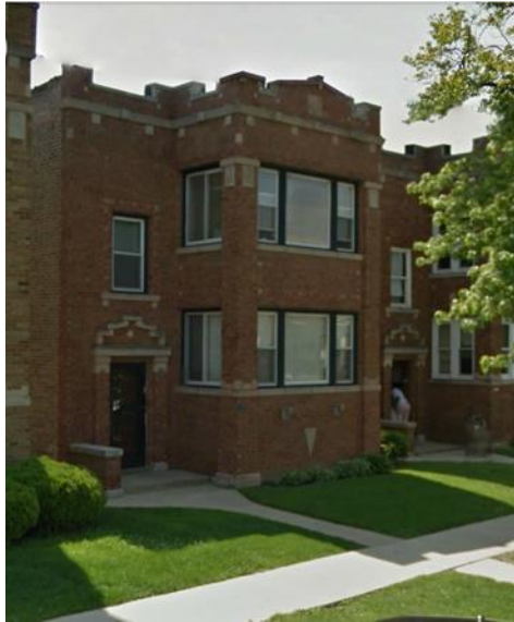
The house today with modern window replacements.
