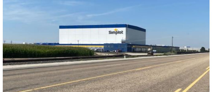
Fig. 12. Simplot plant in Caldwell. Shipping and receiving via rail and truck.
