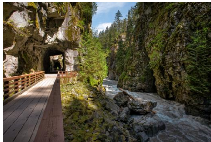
Othello tunnels prior to November 2021 storm. BC Parks photo
