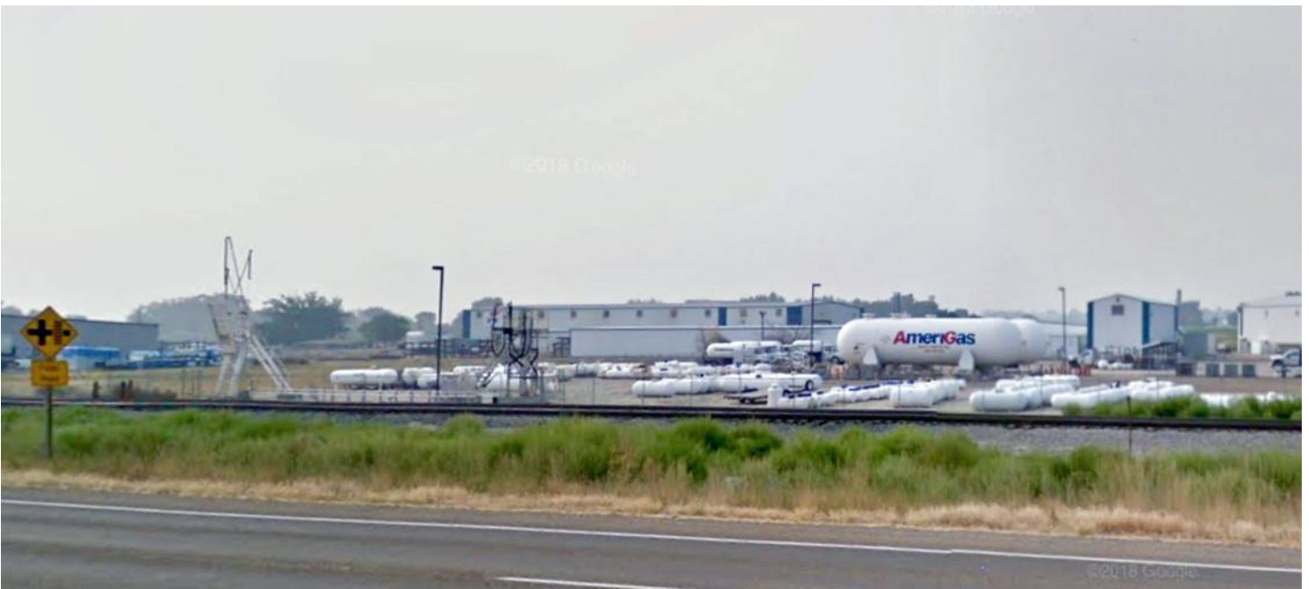
Fig. 9. AmeriGas propane facility between Caldwell and Wilder on ID 19. Google Image
