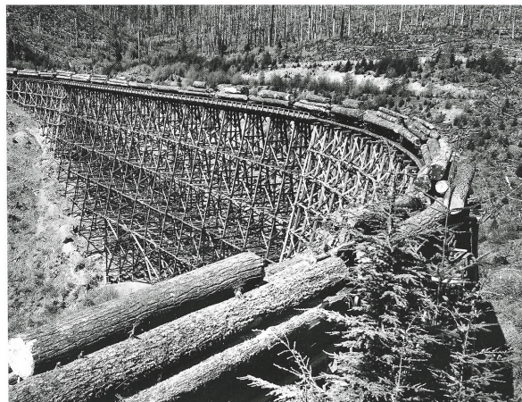
Baird Creek Bridge (Courtesy of Timber Times Vol 49 August 2011 - Weyerhaeuser Archives, No. B07-0013-2) At 1300 feet long and 235 tall, this was billed as one of the world's largest wood bridges. Located in the Kalama River Basin east of Longview, Washington.
