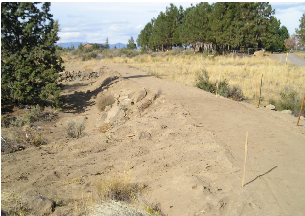
New right of way settling in
